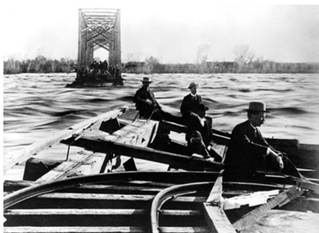
Tempe Railroad Bridge Washed out by Flood (Herb and Dorothy McLaughlin Collection, Arizona Collection, ASU Libraries)
