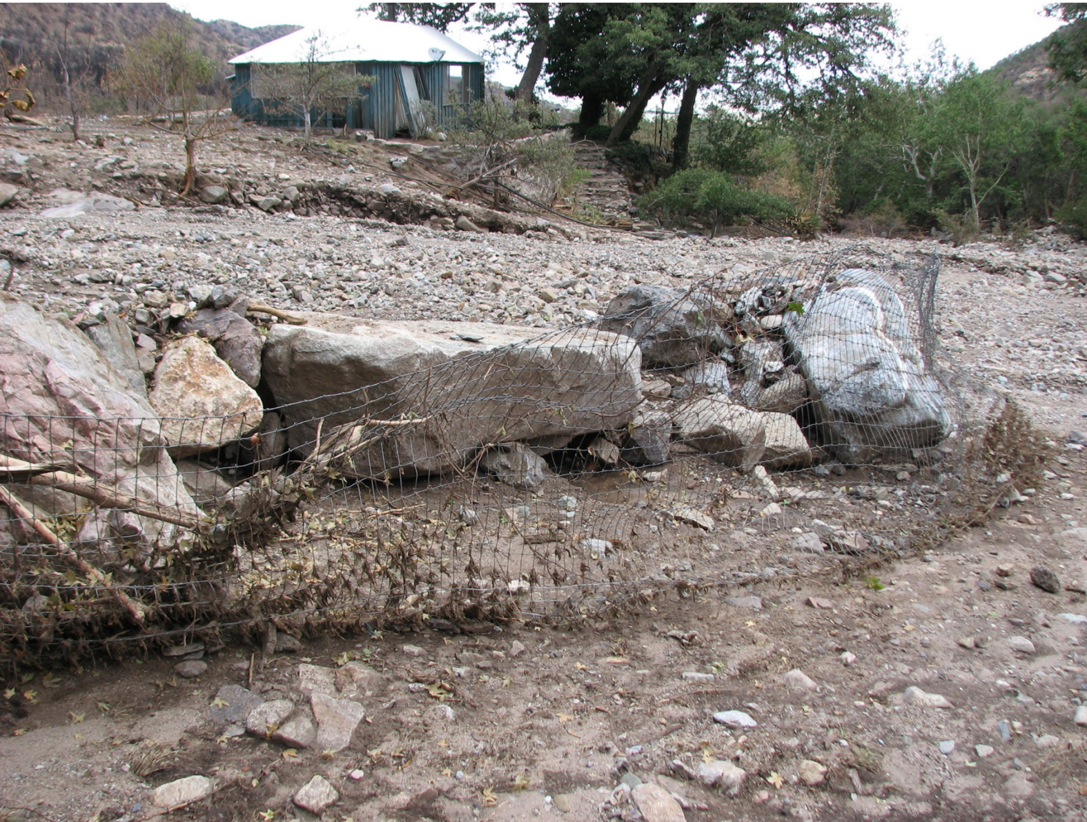
2011 Monument Fire Miller Canyon/Beatty's Debris-flow deposits in Foreground, flood damaged Cabin in background.
