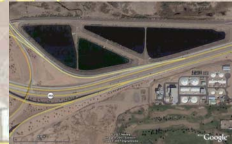
Recharge basins at the Northwest Water Reclamation Plant
